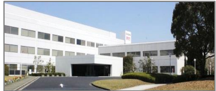
Medical Development Center (Shiga Yasu Plant)
