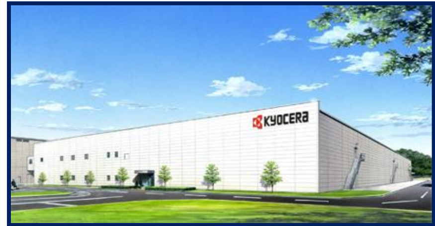
Second facility at the Kyoto Ayabe Plant of Kyocera SLC Technologies Corporation
