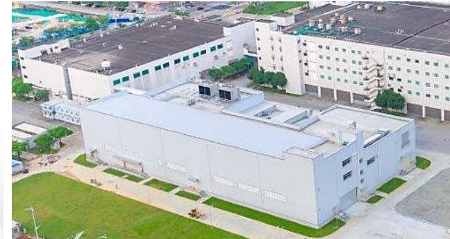
10 th factory in China (No. 2 factory for new OPC* drums)
