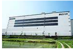
■ Kyocera Document Solutions Inc. Hirakata Plant (60kW) (introduced in FY2006)
