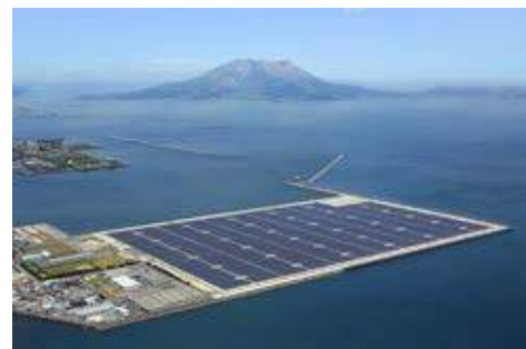
Kagoshima Nanatsujima Mega Solar Power Plant (approx. 70MW), Kagoshima Prefecture, Japan
