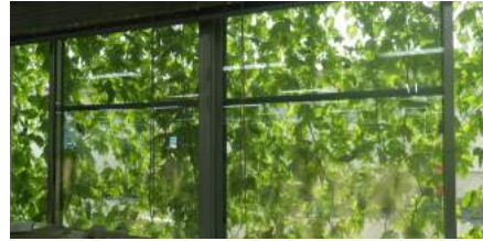
Green Curtain seen from indoors (Shiga Gamo Plant)
