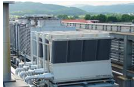
High-efficiency modular chillers
