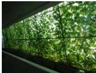
Green Curtain seen from indoors (Shiga Gamo Plant)
