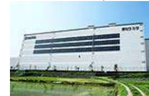
■ Kyocera Document Solutions Inc. Hirakata Plant (60kW) (introduced in FY2006)
