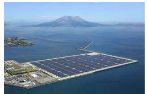
Kagoshima Nanatsujima Mega Solar Power Plant (approx. 70MW), Kagoshima Prefecture, Japan
