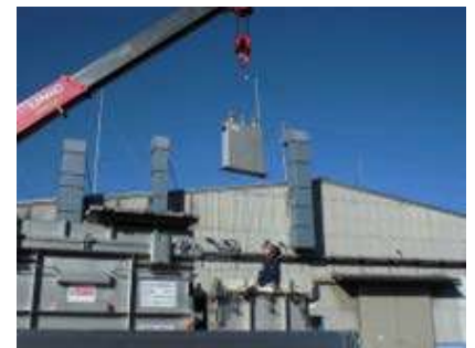
PCB waste load-out work (Tochigi Moka Office)
