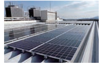
■ Kyocera Document Solutions Inc.'s Tamaki Plant (50 kW) (introduced in FY2011)
