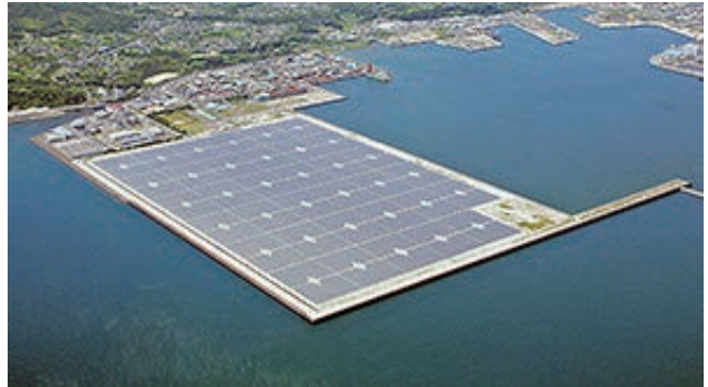
Kagoshima Nanatsujima mega-solar power plant
