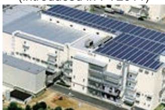
■ Shiga Yokaichi Plant (457 kW) (introduced in FY2006, expanded in FY2011, FY2012 and FY2013)
