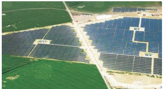
Solar power plant in Cigliano, Piedmont, Italy
