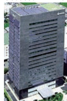
■ Head Office (214 kW) (introduced in FY1999)
