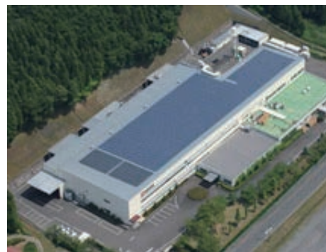
Solar power generating system installed at the Fukushima Tanagura Plant (230 kW)
