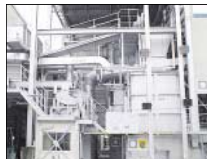
Intermediate processing complex facility (Kagoshima Sendai Plant)
