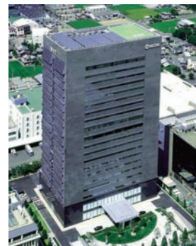
Installed 1,896 solar cell modules on the roof and the south wall
